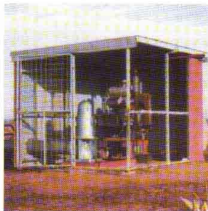
Typical farm installation, Batescrew angle gear drive pump, 150 litres/second, 22 metre 41kw. Deniliquin, New South Wales.
