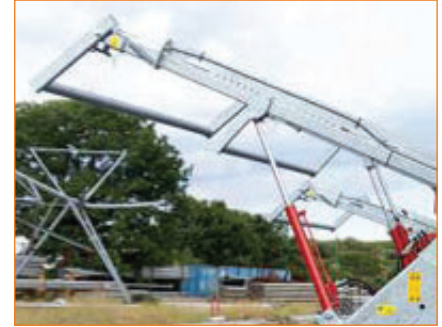
Lifting of the trolley
